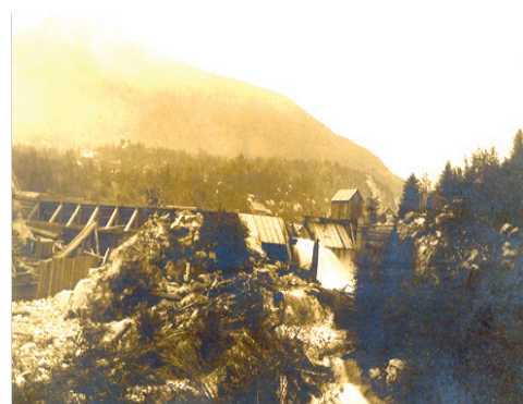
The hydro electric generating plant at Cottonwood Falls was built in 1895-1896 and was the first hydro generating station in BC. Photo, circa 1898, courtesy of Touchstones Nelson.
