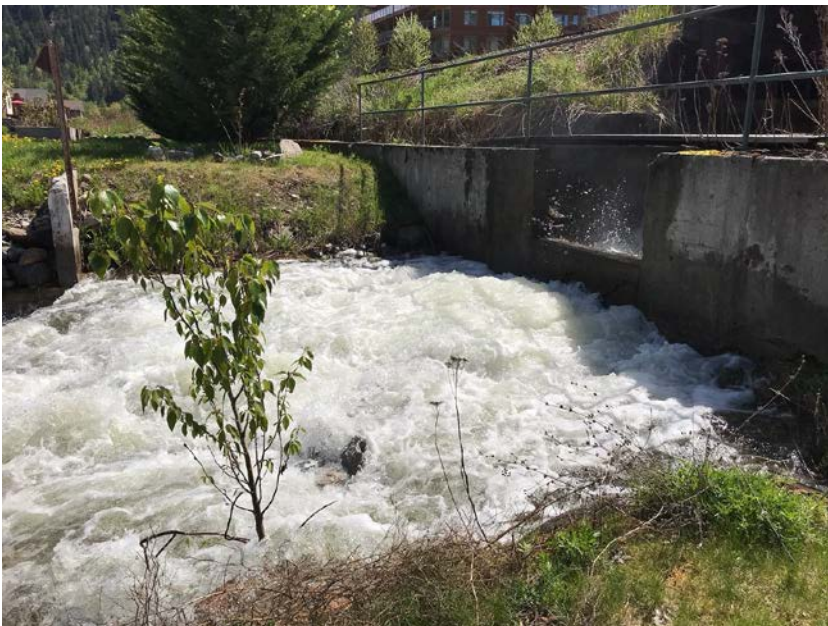
Anderson Creek in Fairview
