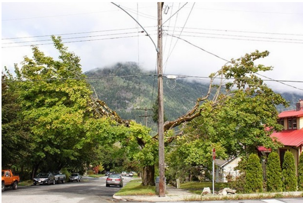
Figure 4. Example of "V" cut trimming in Nelson
