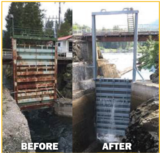
Replacement of forebay head gates
