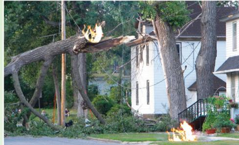
Trees making contact with electrical lines can start a fire. Note the fire on the grass and on the tree that is laying on the power line.
